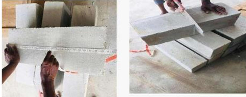
Figure2.3. cutting the AAC blocks in half.
